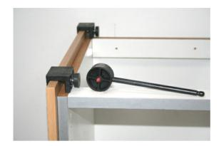
Attach clamps as shown and make sure that you have no daylight between the Clamp top and the end panel top
